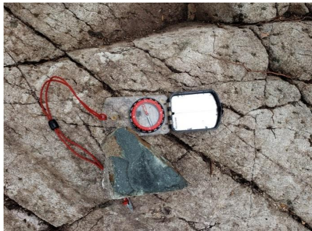
Gabbro exposed at Lot 25 Trenches; note strong joint set oriented 140° and 110°
